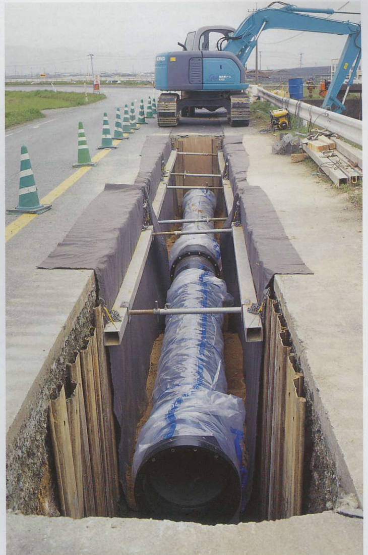
Polyethylene sleeves being used to protect Ductile Iron Pipe.
