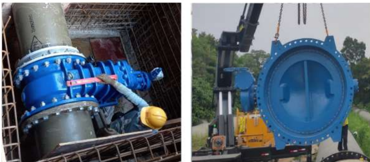
Gate Valves &amp; Swing Check Valves at site
