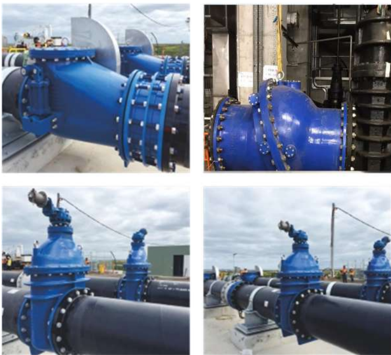
Gate Valves &amp; Swing Check Valves at site
